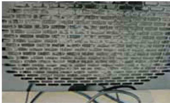
Figure 50: Dirt on the condenser 2
